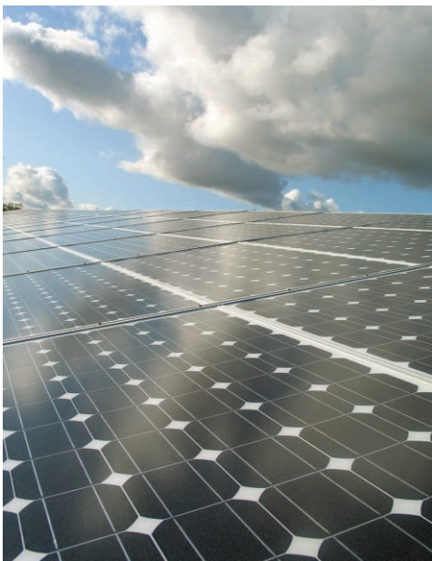
35KW grid connected solar roof system in Dunkirk, France
