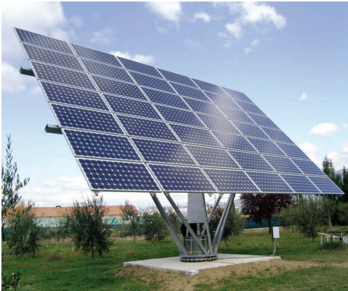
7.6KW grid connected photovoltaic tracking system in Italy
